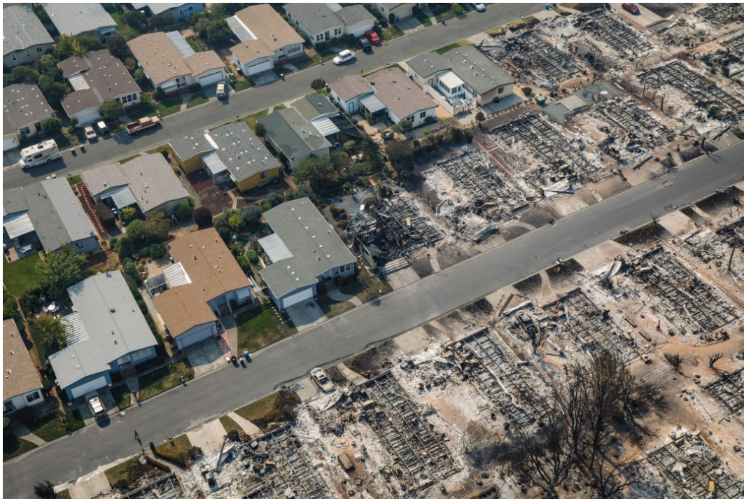
Some homes in Coffey Park were undamaged in the 2017 Tubbs fire, while others were destroyed. (Marcus Yam / Los Angeles Times)
