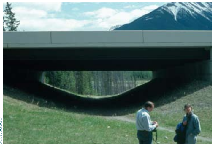
Underpasses designed for wildlife can provide for safe passage and link habitats.
